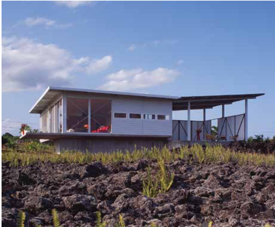
Above, Lavaflow 2, Steely's own house in Kalapana where he lives half of the year, seems to float above a lava field, part 1960s glass house and part Island-style bungalow.
